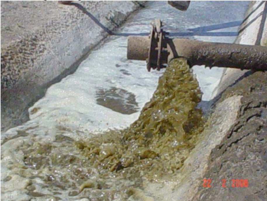
Figure 8 – Discharge to Irrigation Channel
